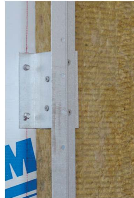
Generic adjustable back to back L-angle clips.
