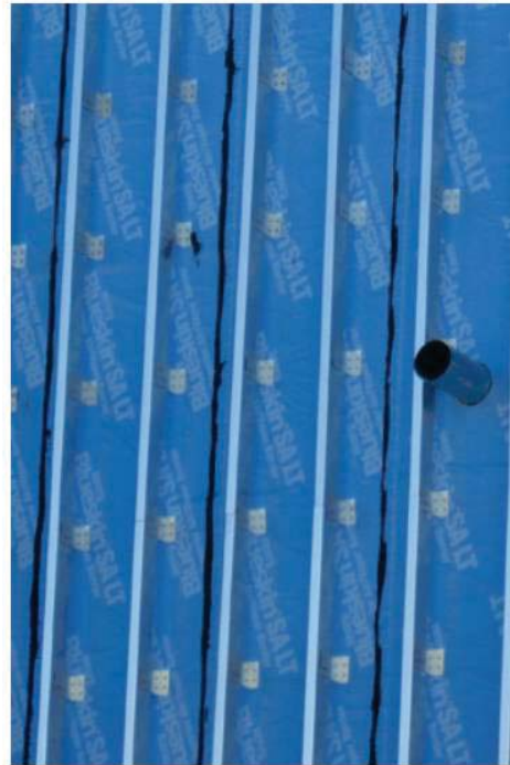
Intermittent galvanized steel clips with vertical girts.
